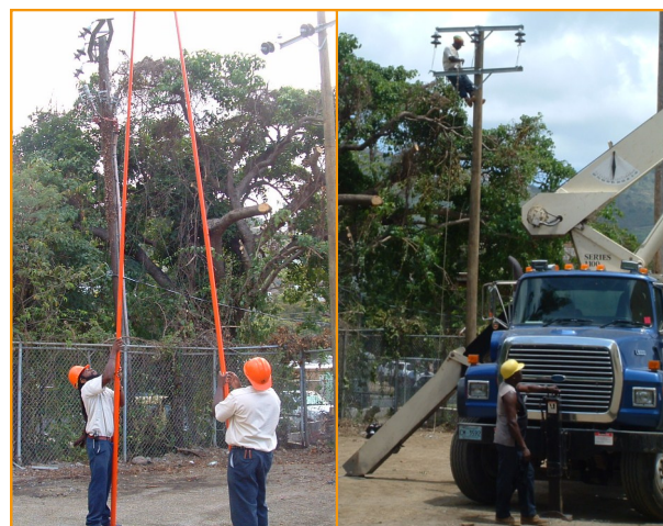
Linesmen measure voltage levels
